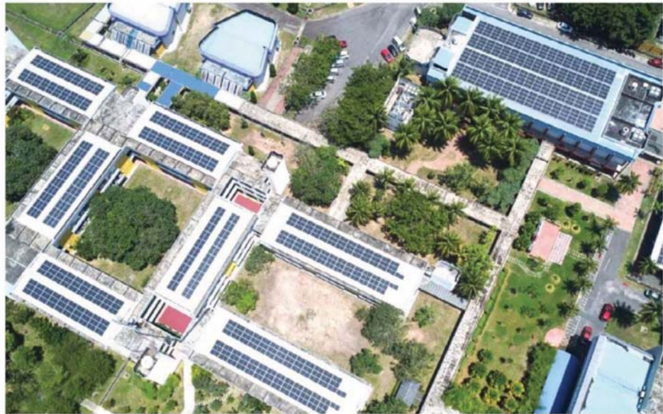
An aerial view shows the solar panels installed on buildings at the campus. — Bernama photo
