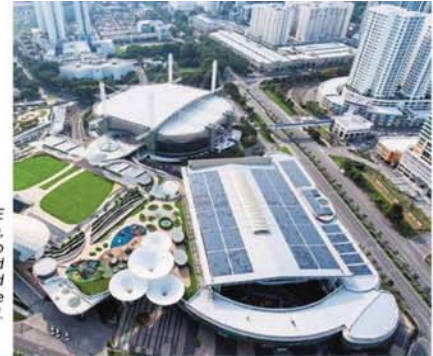
Setia SPICE Convention Centre, Penang is said to be the first hybrid solar-powered convention centre in the world.
