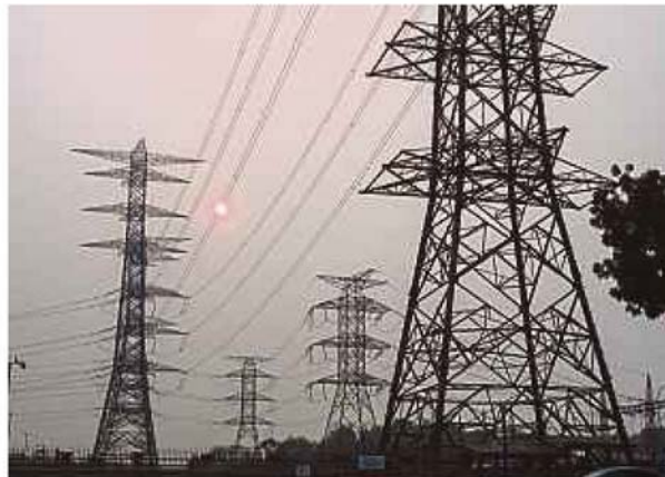
The contract is valued at RM568.2 million. NSTP FILE PIC
