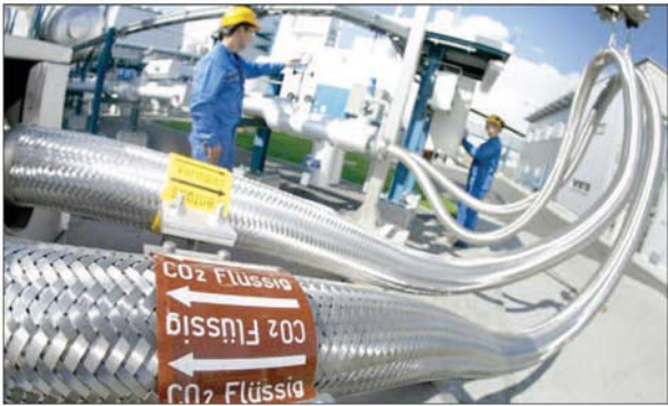
Employees work on pipes carrying liquid carbon dioxide at a power station near Berlin, Germany. (AFP)
