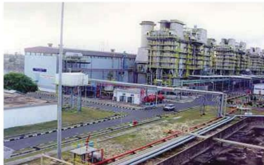
Tenaga Nasional Bhd says the repowered Sultan Ismail Power Station in Paka, Terengganu is projected to generate an average RM250 million per year in earnings before interest and taxes.
