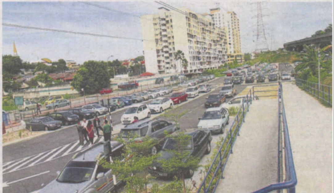
Aside from the 320 parking bays, the project also involved 25 additional parking spaces in a separate lot for nearby residents of the Sri Aman flats. — SHAARI CHEMAT/The Star
