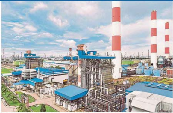
In Singapore, Maybank, DBS and OCBC jointly extended a S$500 million transition loan to YTL PowerSeraya.
