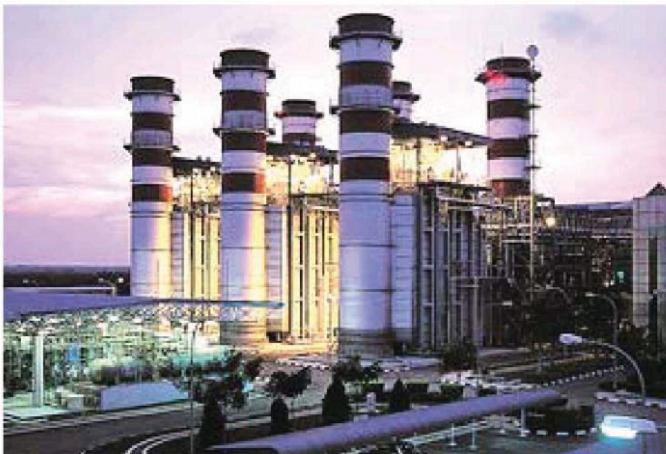
The project's pre-funded contingency sum and construction cost savings to-date provided sufficient liquidity to enable Edra Energy meet their financing obligations due in January 2022 under its RM5.085 billion Sukuk Wakalah, which has a maturity date on 2038 and rated AA3/Stable.
