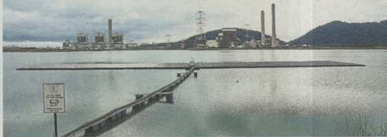
For floating solar, TNB made use of its ash pool at Sultan Azlan Shah Power Station to construct its pilot floating solar plant with an installed capacity of 105.12kW
