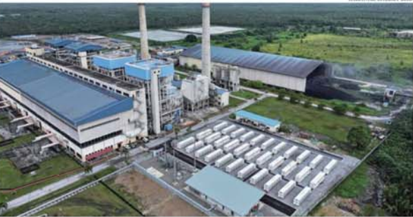
Battery storage system located in Kuching, Sarawak
