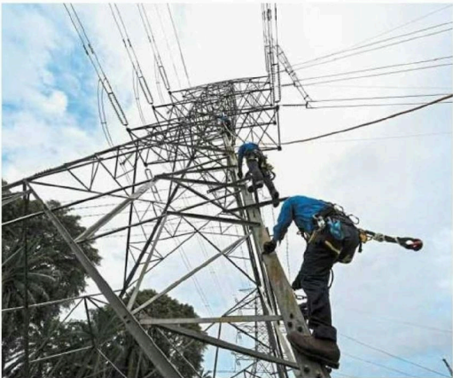
Technicians climbing a high voltage tower to carry out a tower-top inspection as part of scheduled maintenance work in Skudai, Johor Baru.
