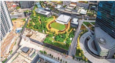
An overview of Taman Bandar TRX @ TRX City Park. — GDP Architects & Oculus
