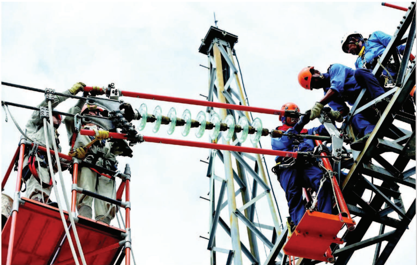
The hot team (left) examining the tempered glass plate insulators, assisted by the cold team perched upon a gantry structure at Bukit Beruntung substation. — Pictures by Azneal Ishak
