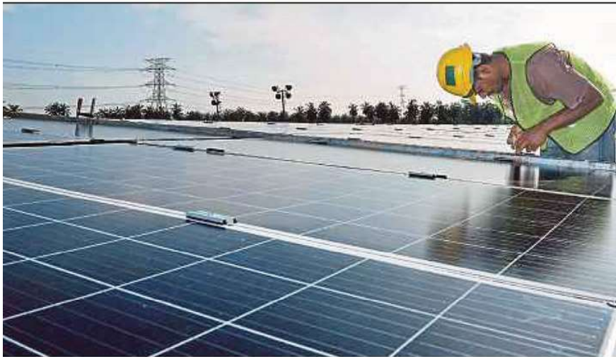
Tenaga Nasional Bhd's large-scale solar project in Kuala Langat, Selangor, which has 230,000 solar panels and 10km of 132kV power and fibre optic underground cable, is Malaysia's largest to date.
