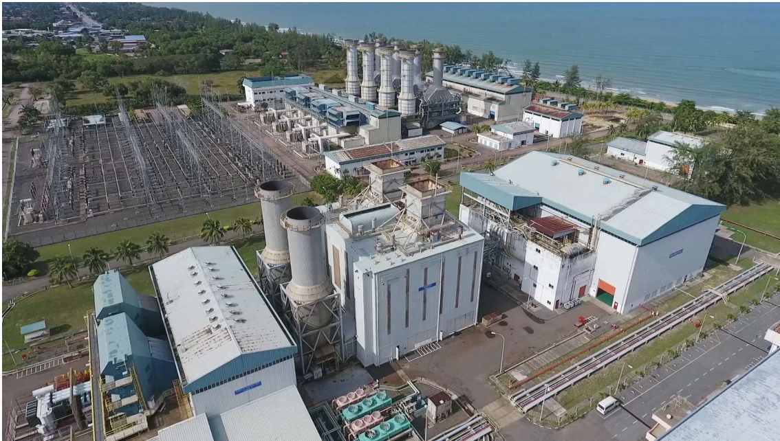
PHOTO 2: The Sultan Ismail Power Station (SJSI), world's largest combined-cycle power station in 1987, officiated by the late Sultan Mahmud Al-Muktafi Billah Shah, was officially decommissioned on December 31, 2019.
