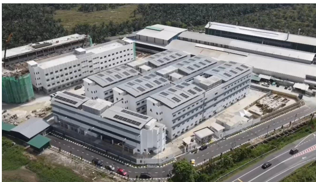
Tenaga Nasional Berhad (TNB) and its wholly-owned subsidiary, GSPARX Sdn Bhd signed a Supply Agreement with Renewable Energy (SARE) with Central Medicare Sdn. Bhd (CMSB) for the installation of solar photovoltaic (PV) facilities at the CMSB factory and hostel sites in Teluk Intan, Perak, with a total capacity of 6.039 MWp.
