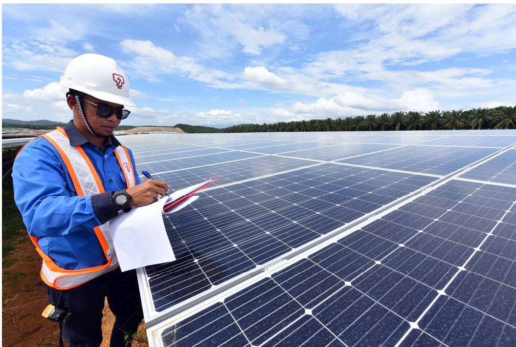
PHOTO 2 - A TNB staff checking the solar photovoltaic panels at the Bukit Selambau large scale solar project, located 25km from Sungai Petani, Kedah. The project on the 50-hectare land is 84% complete.
