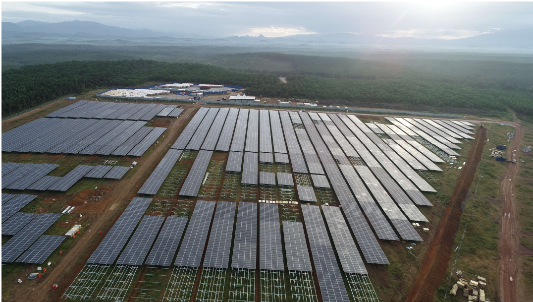
PHOTO 1 - Tenaga Nasional Berhad's (TNB) second large scale solar project in Bukit Selambau, Kedah, involves the installation of 134,880 solar photovoltaic panels that can generate up to 30 megawatt.
