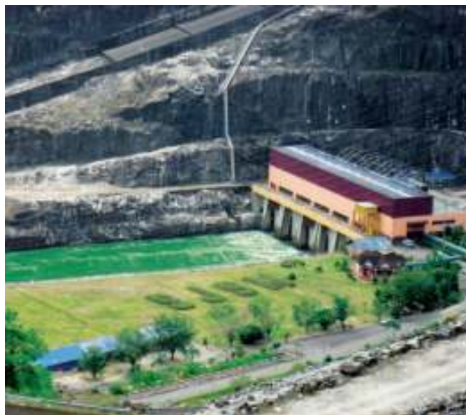
Above: Sultan Mahmud Power Station, also known as Kenyir Dam, is capable of generating an average annual energy output of 1,600GWh. It serves the dual purpose of providing hydroelectric power and serving as a flood mitigator.
