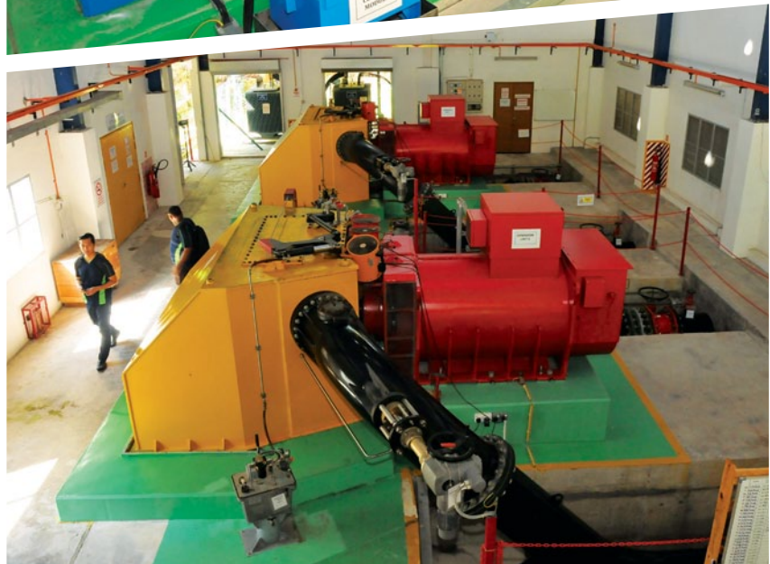
Above right: This 2MW generator was installed at the plant in 2015, stretching its total capacity to 6MW.
