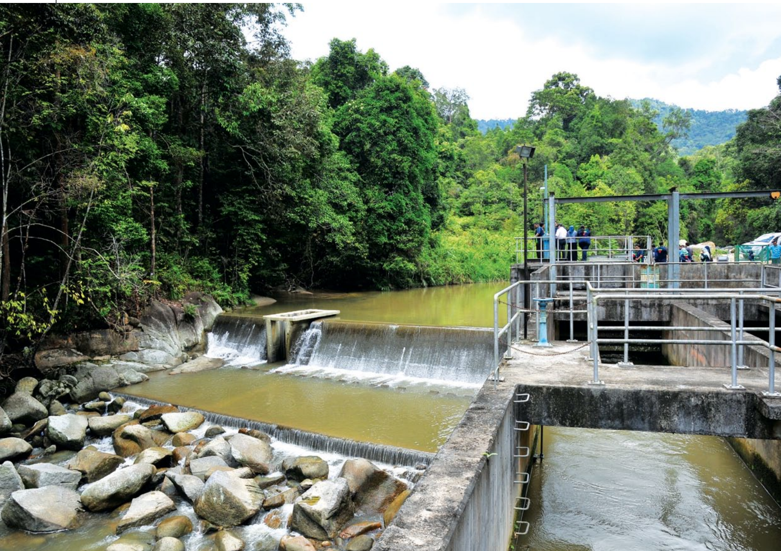
Traversing across the river, the weir helps to direct water into the intake plant (right).
