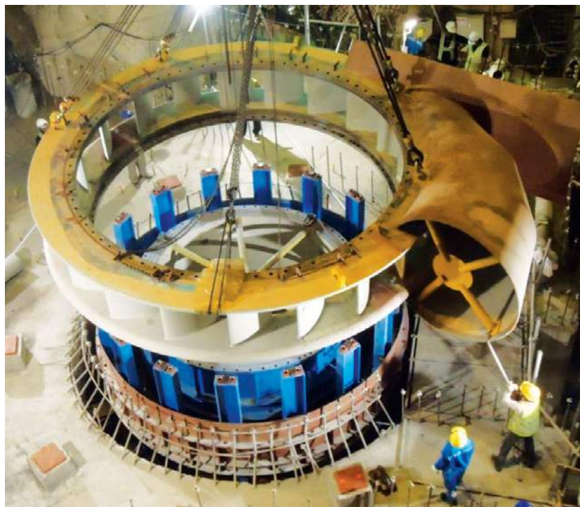
A bird's eye view of the components of the hydropower turbine which can generate 125MW of electricity.
